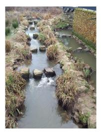
The sign explains it to us: a weir here ensures that the water is high enough to supply the canal (because water always runs "downhill", and the water in the canal is not always lower than the Dijle!). That difference in height can be a meter and a half, which is a bit much for fish... That's why we have a fish ladder: 23 small steps of 7 centimeters which the fish can take or "bridge" (without bridge).
